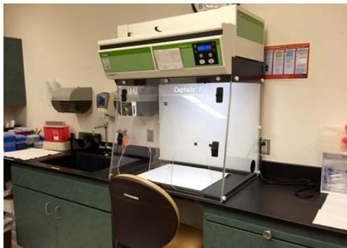
Fume Hood for Hazardous Chemical Handling and Stool Preps
